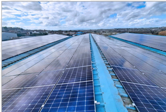
Over 600 solar panels were installed across two sites, generating over 230,000 Watts Peak.
